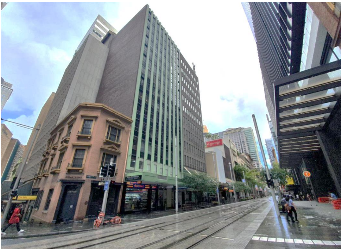
Figure 2-14 The Former Skinners Family Hotel at 296 George Street and adjacent office buildings
