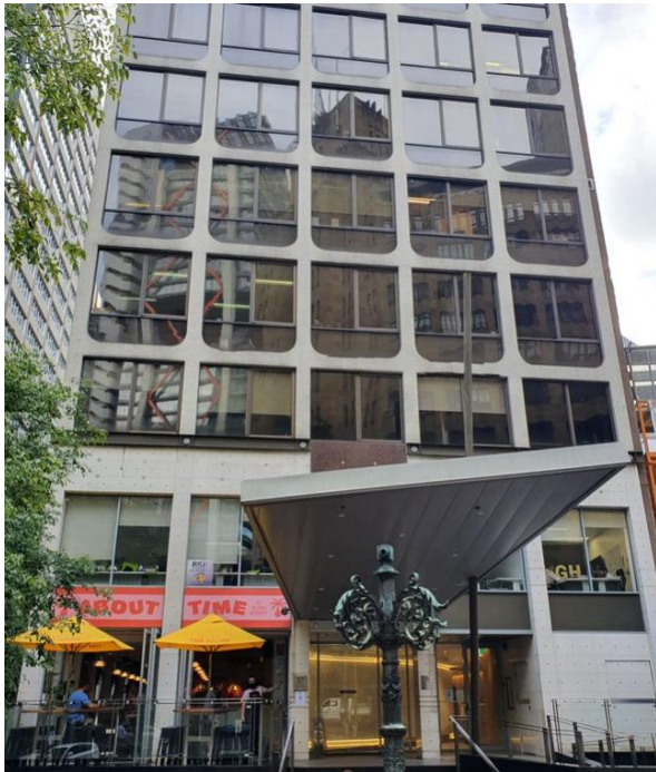
Figure 2-5 Existing office building at 37 Bligh Street
