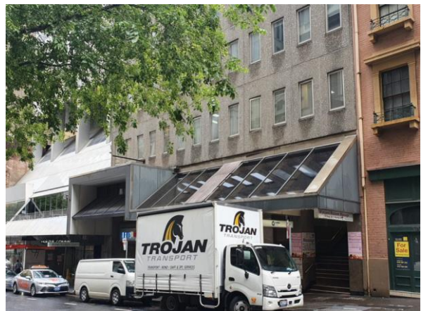
Figure 2-13 Existing commercial building at 5 Hunter Street
