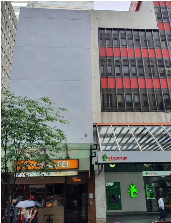
Figure 2-10 Existing commercial buildings at 312 and 314-318 George Street
