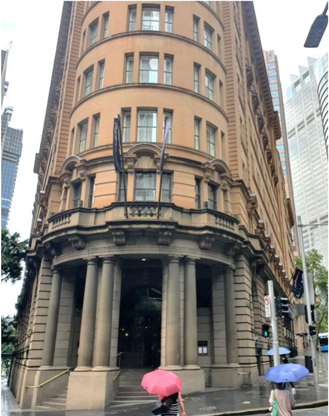
Figure 2-21 Radisson Blu Plaza Hotel at 27 O'Connell Street
